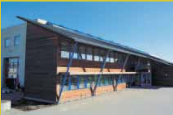
STEMA/PEDAX Headquarter – Denmark
