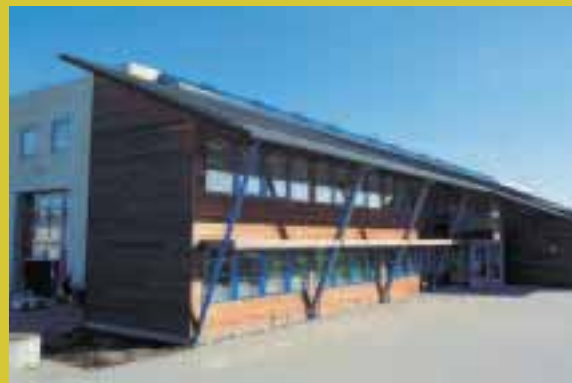
STEMA/PEDAX Headquarters – Denmark
