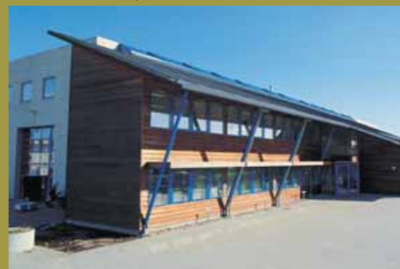
STEMA/PEDAX Headquarters - Denmark
