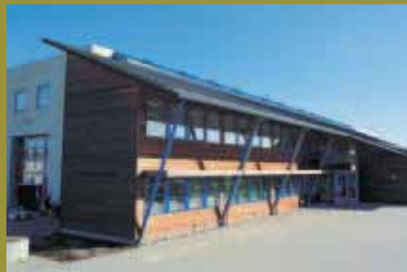
STEMA/PEDAX Headquarters – Denmark
